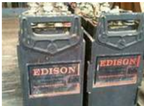
Gambar 10.10: Baterai Nikel Besi (bing.com/images-diakses 2024)
