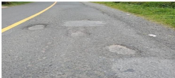
*Gambar 2. 9 Lubang (Potholes)*
