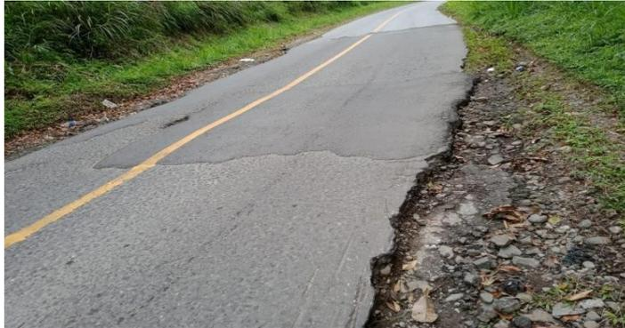
Gambar 2. 8 Tambalan (Patching end Utiliti Cut Patching)
