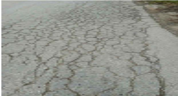
*Gambar 2. 5 Retak Kulit Buaya (Aligator Cracking)*
