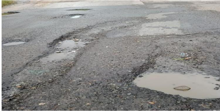
*Gambar 2. 6 Pelepasan Butiran (Weathering/Raveling*
