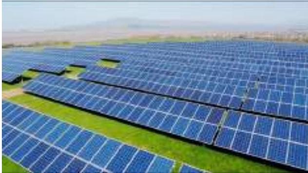
**Gambar 3.7:** PLTS Ground-Mounted (ESDM, 2019)
