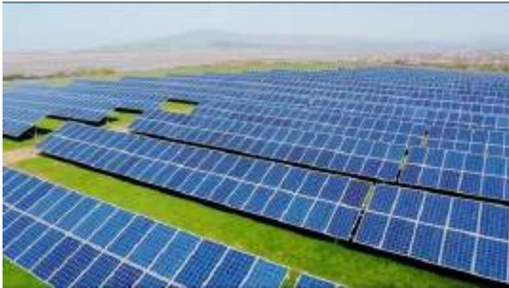
**Gambar 7.4:** PLTS Ground-Mounted (ESDM, 2019)
